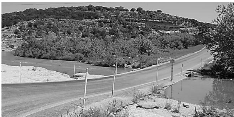
FIGURE 8. Low-water crossing on a Texas highway. Image copyright TexasFreeway.com. Reprinted with permission.
