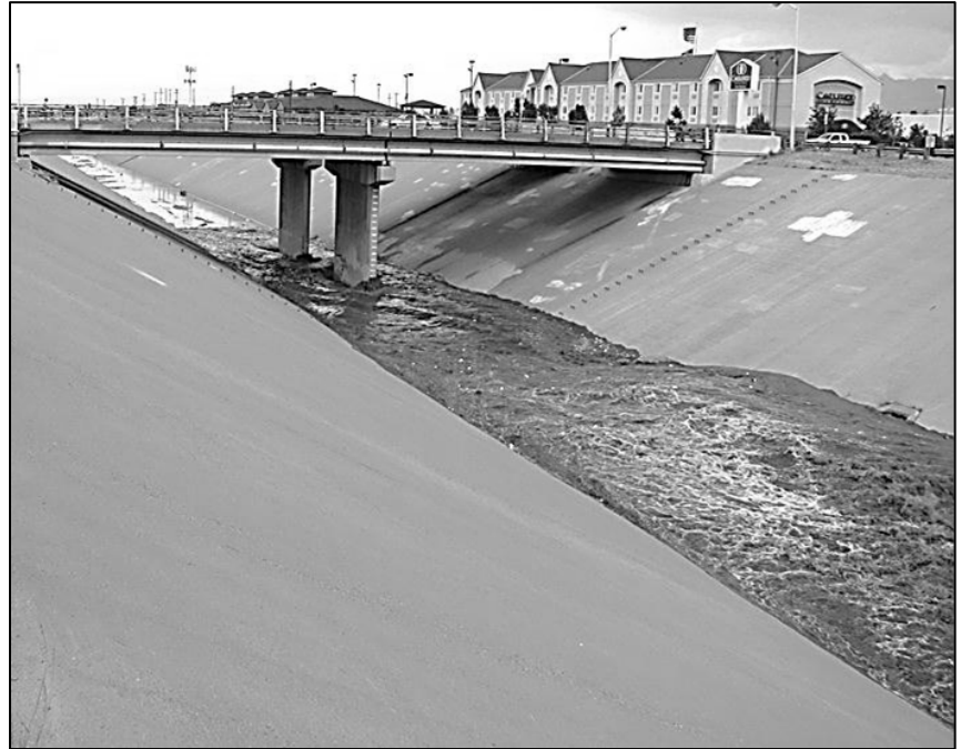
FIGURE 7. Storm surge within a concrete flood control channel in Albuquerque, NM. Downstream the water is six inches deep, upstream it is nearly five feet deep, with the leading edge moving 20-30 mph. Photo taken June 23, 2009. Image courtesy of Albuquerque Metropolitan Arroyo Flood Control Authority.
